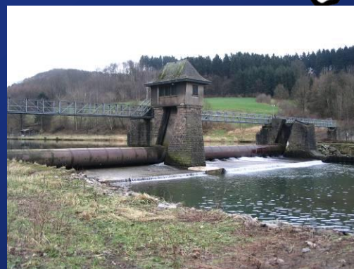
Wehr Wintersohl, km 47+400
